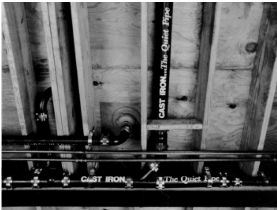
Figure 1—Cast Iron in Residential Application.
